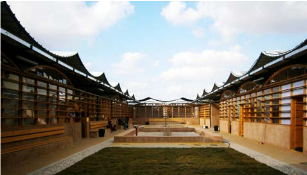
Fig. 3. Courtyard in Um al Nasser children's center. Rainwater is collected by gutters, deputed and then stored in an underground tank. Design by: ARCò, & MCA. Promoted by: Vento di Terra ONG.
